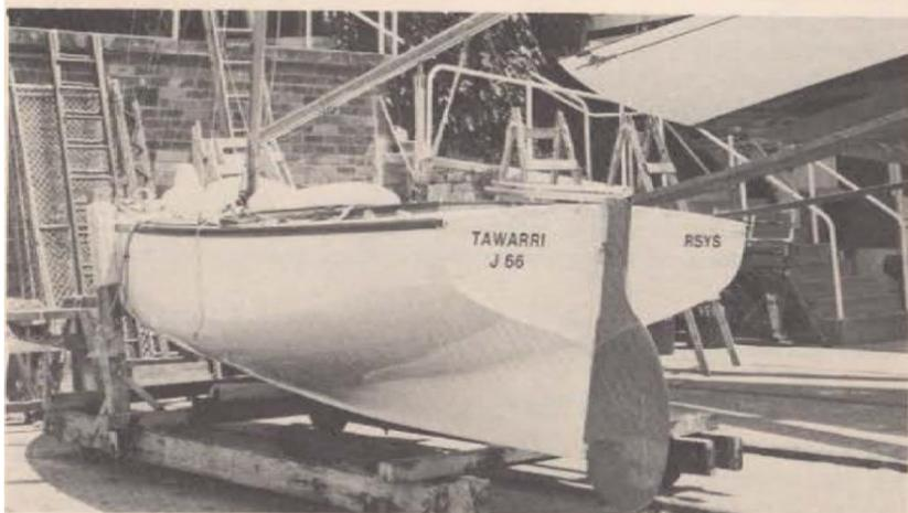
*Timber Jubilee showing hull lines, skee and rudder.*
